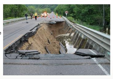
As Walleser exited the bridge span his vehicle entered an area of the roadway that had washed out causing his vehicle to fall into the river. Walleser's vehicle was completely submerged. The highway surface appeared to have been under-cut due to the high water; ultimately, causing the highway surface to erode and fall into the river. There was a witness who was a quarter mile behind Walleser who contacted the Sheriff's Department.
